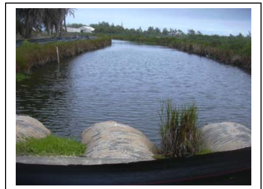
Pipes direct runoff from the industrial sector of Kahului and transport water under the road to the drainage canal in the direction of the VIP property (below).
